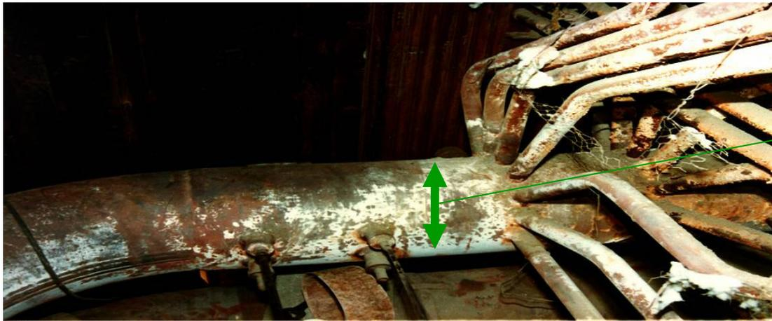
**Stretching of the material because of temperature gradients lead to lifetime reduction**
